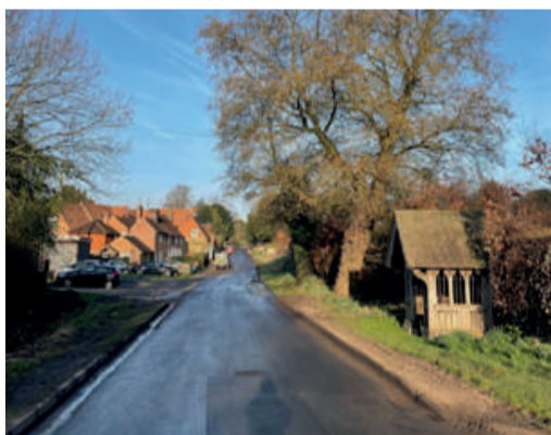
The Pump House
