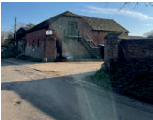
Atheralls Farmhouse Barn
